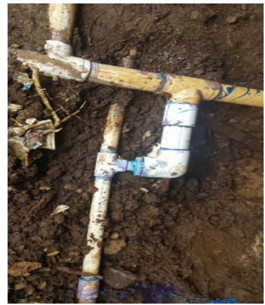
Landscaping repaired a damaged irrigation pipe located at the Alii lawn.
