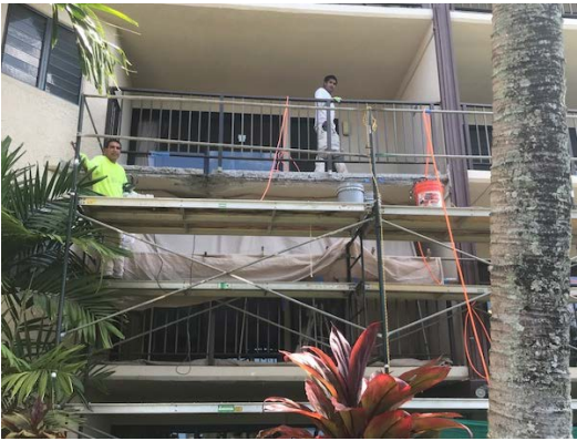
JD Painting completed spalling work on unit 3111, 3112 & 3212 spalling.
