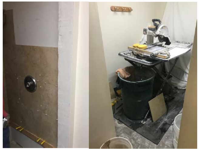
Lihue Drapery & Flooring started work on the Roof Top Center Shower.
