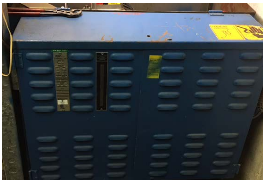
Banyan East elevator hydraulic tank leaked as it was rusty. Terry has ordered the replacement tank.
