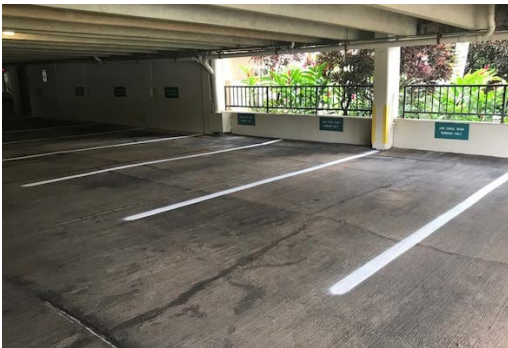
Engineering started to re-stripe the parking garage stalls.
