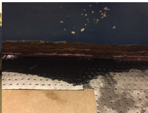
Banyan East elevator hydraulic tank leaked as it was rusty. Terry has ordered the replacement tank.
