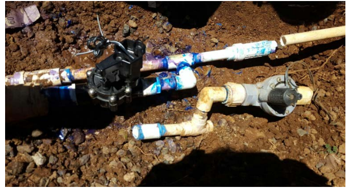
Landscaping repaired a defective sprinkler valve fronting the Coral building.
