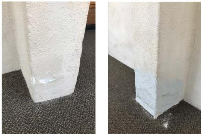
Engineering started to repair the damaged stucco on the Banyan hallways.
