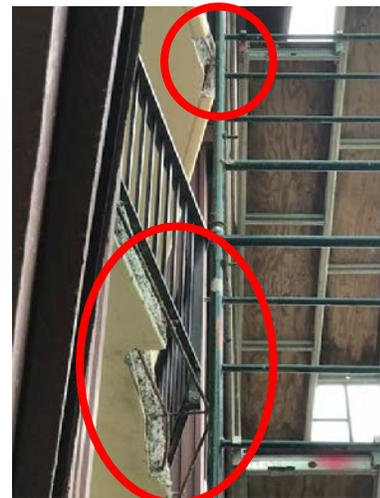
JD Painting repaired the lanai of unit 1308 and 1407. JD identified a crack in unit 1407 lanai and it was added to the scope of work.
