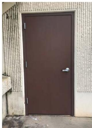
Engineering replaced the first-floor garage door with a lighter metal door.
