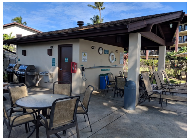
Engineering painted the walls of the Alii pump room.
