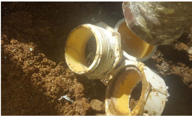
Cabreira Plumbig repaired the main water line to the Coral building. The fitting cracked inside the cement foundation.
