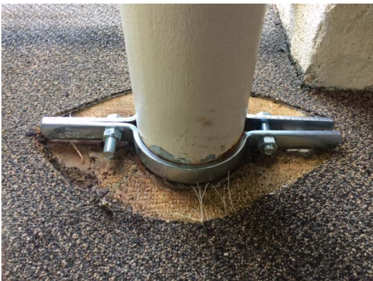
Protech Fire replaced the rusted dry standpipe clamps at Banyan building. Engineering is rust treating and painting the brackets red, for visibility.
