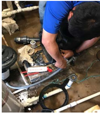
Engineering replaced the cracked housing of the Alii pool pump.
