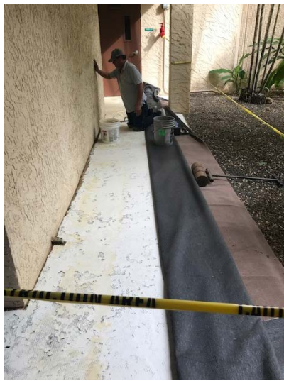
Lihue Drapery and Flooring installed the sample Marine outdoor carpet on the first floor of the Coral building.
