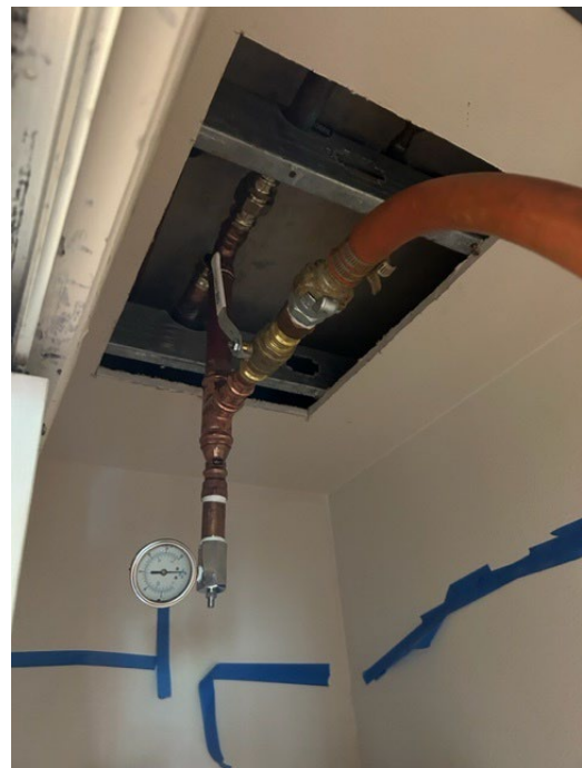
No Ka Oi Plumbing attempted to epoxy coat the main water line for the 2105 stack as we have a leak in the main between 2303 & 2403. We were unable to repair, so they will need to return to try and isolate it even more.
