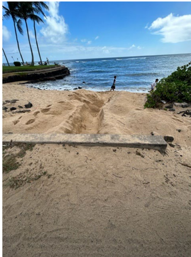
Landscaping cleared the culvert prior to the Tropical storm Hone & Hurricane Gilma to prevent flooding of the parking lot.
