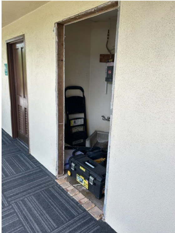
Engineering replaced the housekeeping service room entry door frame as it was rusted causing the door not to shut properly.
